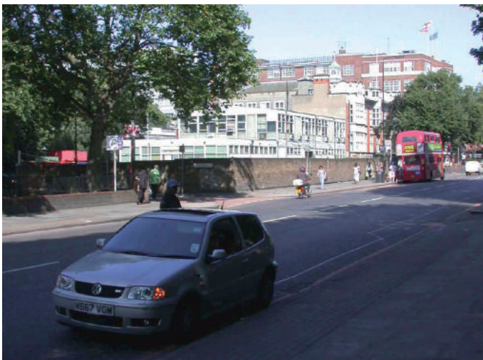
View of the existing building looking east down Peckham Road
