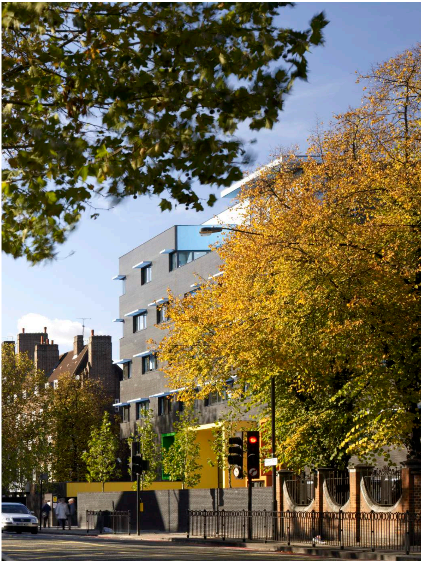
The setback from Peckham Road matches the adjoining buildings
