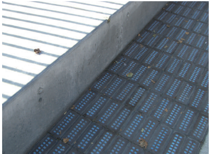
Filling the bricks with Terrazzo forms a coloured "carpet" laid in front of seating at the main entrance.
