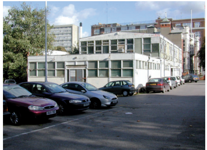
The Existing Southwark Council Administration Building on the site in 2001
