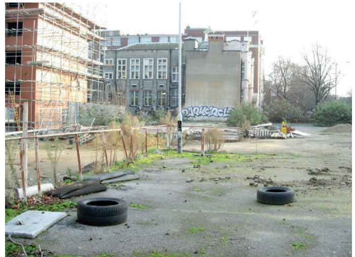
The existing building was demolished in 2004 - shown here is the site in 2005
