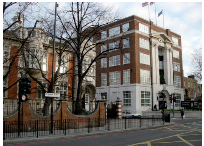
Southwark Town Hall and offices lie immediately adjacent. Both are listed buildings, which set the height of the building's eastern end.
